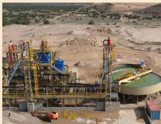
Overview of the wet portion of a fracturing sand plant designed and provided by Outotec
